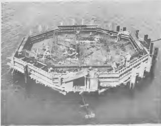
LAGOON BIGGEST over-water concrete operation took place June 23 at No. 3 Finger Pier's turning dolphin where 289 cubic yards of concrete were poured non-stop. E. OPERACION di concreto ariba awa mas grandi na Lago a tuma lugar Juni 23 na e dolfin gigante di No. 3 Finger Pier unda 289 yarda cubico di concreto a worde basha.
